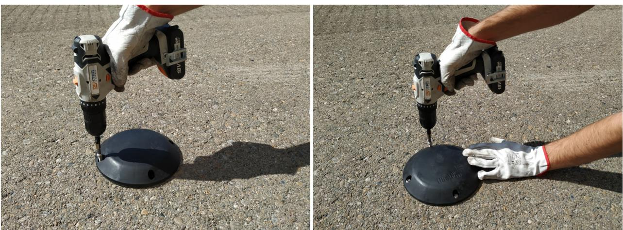
Figure : Screw the node
