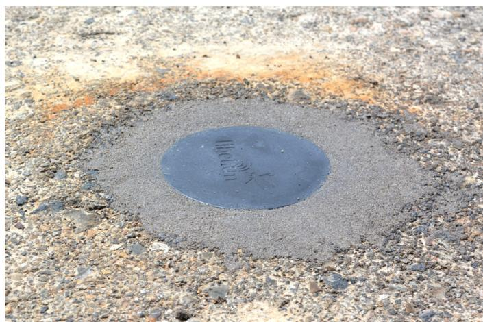
*Figure : Final Epoxy application*
